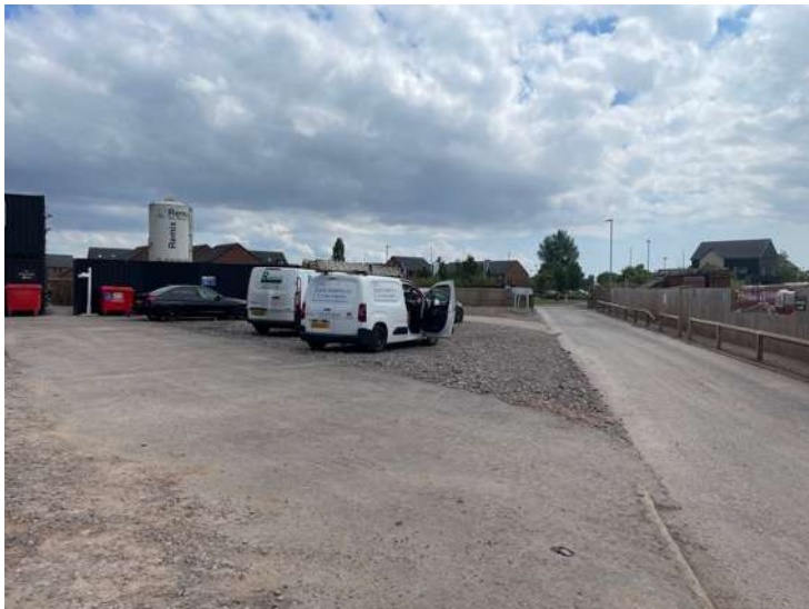
Photo 4: View towards South through zone of proposed retail units and car park 10 th June 2024.
