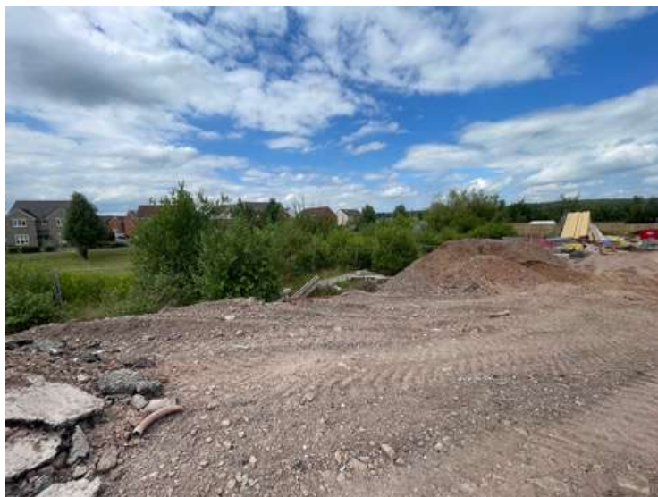
Photo 1: View from proposed Lidl site area towards North/North-West and proposed Nursery from centre of site 10 th June 2024.
