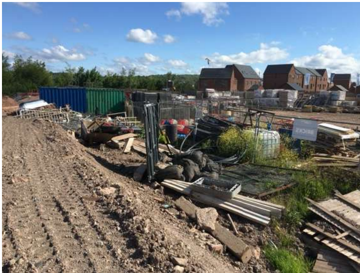
Photo 3: View from location of proposed Nursery Unit car park towards North-East over location of proposed retail units 10 th June 2024.
