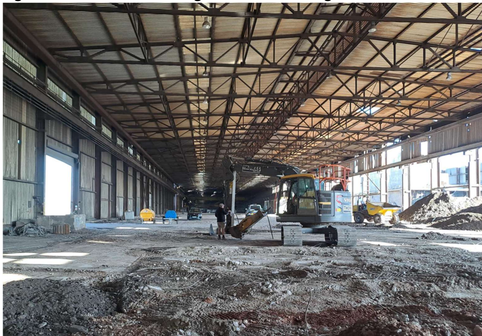
Figure 1: View with the existing steelworks building
