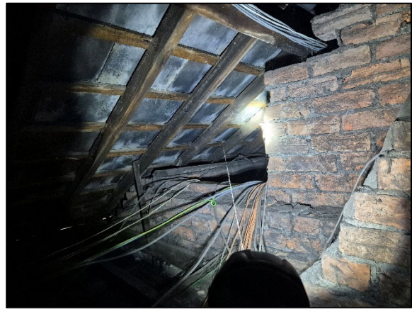
Figure 16 – Light Ingress via Gaps Present on (N) Side of Loft, May Permit Access/Egress for Bats to (N) Section of Loft Interior
