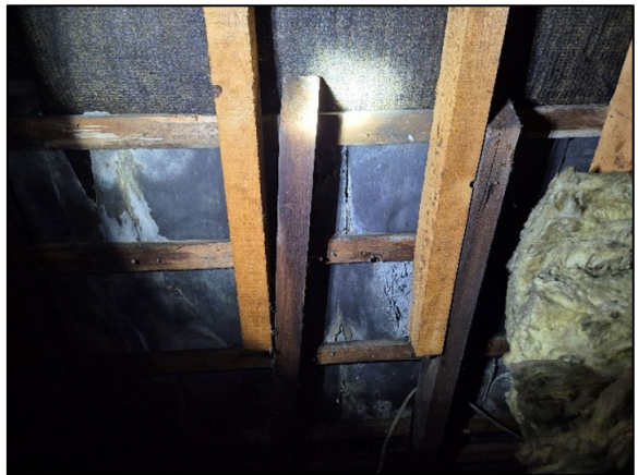
Figure 26 – Detail of Underside of Roof. Although Most of the Roof Tiles are Overlaid Directly onto Battens, Some Roof Felt Underlay is Present in Some Areas
