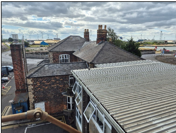
Figure 9 – Roof of MSB in Picture Background
