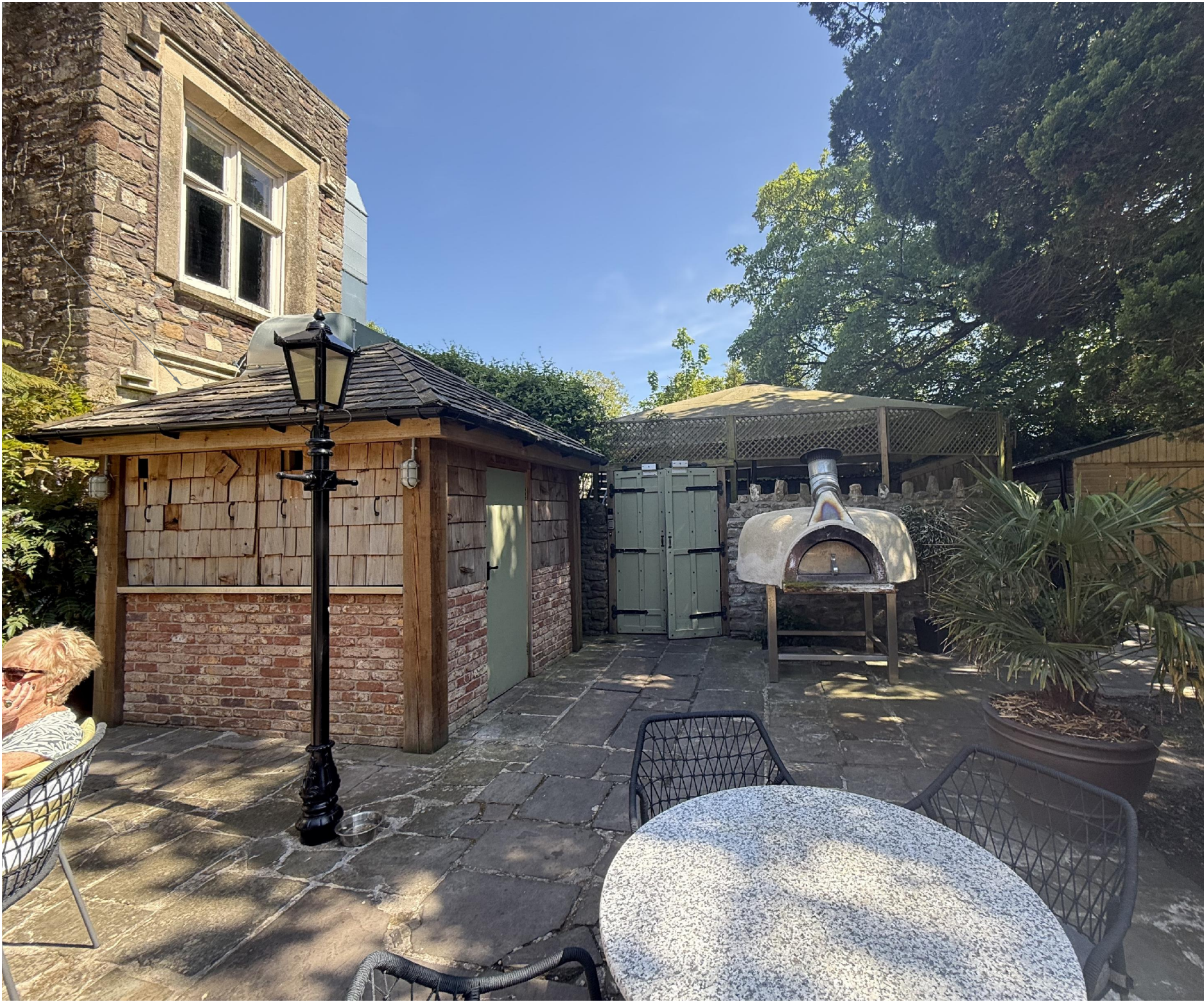
EXISTING LOCATION REFERENCE IMAGE 04 - SHOWING 'PART A' VIEW FROM GROUND FLOOR LEVEL TERRACE/GARDEN
