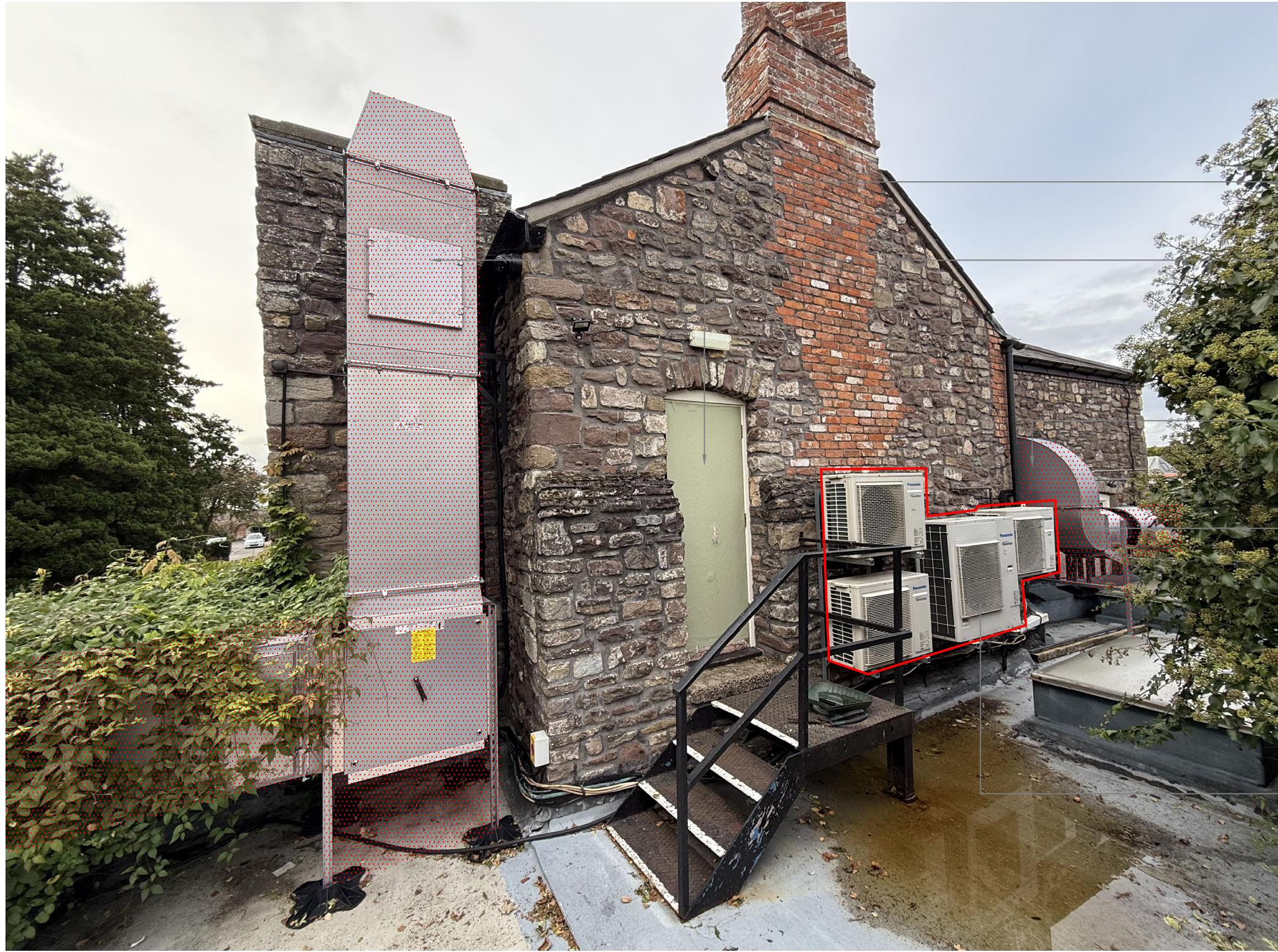
PROPOSED LOCATION REFERENCE IMAGE 01 - SHOWING 'PART A' AND 'PART B' EQUIPMENT LOCATIONS VIEW FROM FLAT ROOF (FIRST FLOOR LEVEL)
