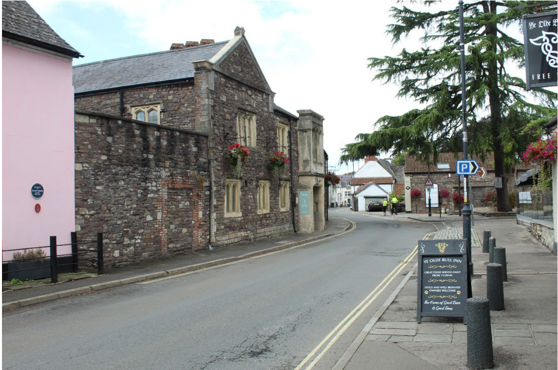
Image EDP A1.1: View of the main elevation of The Priory looking west along High Street.
