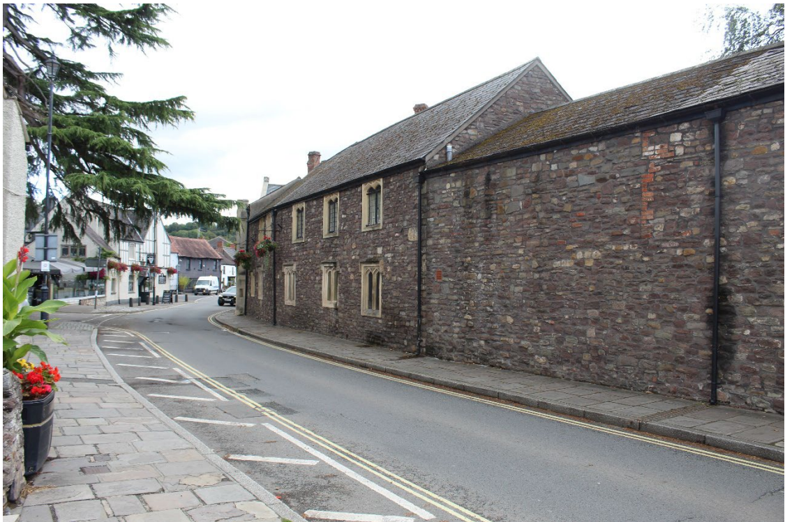
Image EDP A1.3: View of the main elevation of The Priory looking east along High Street.
