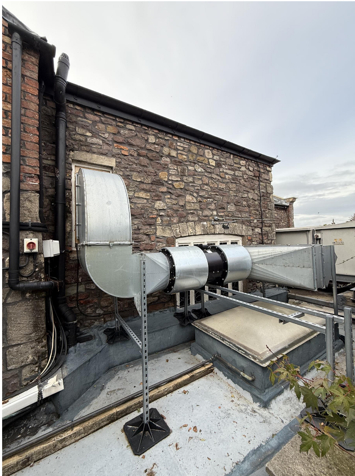
EXISTING LOCATION REFERENCE IMAGE 04 - SHOWING 'PART B' EQUIPMENT VIEW FROM FLAT ROOF (FIRST FLOOR LEVEL)
