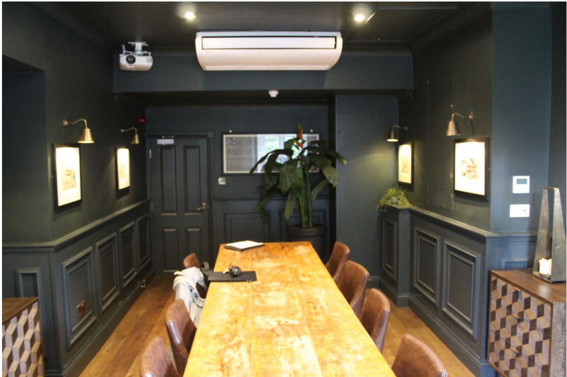
Image EDP A1.12: View of the private dining room on the first floor of the project site, looking north and showing the riser in the north-east corner.
