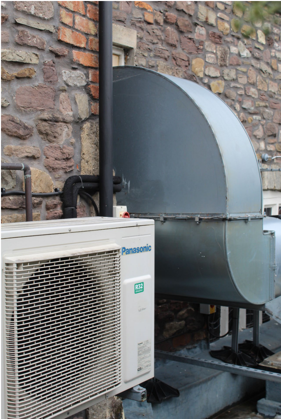
Image EDP A1.19: Close-up of the eastern duct and showing its relationship with the small window opening in the east-facing elevation of the staircase range.
