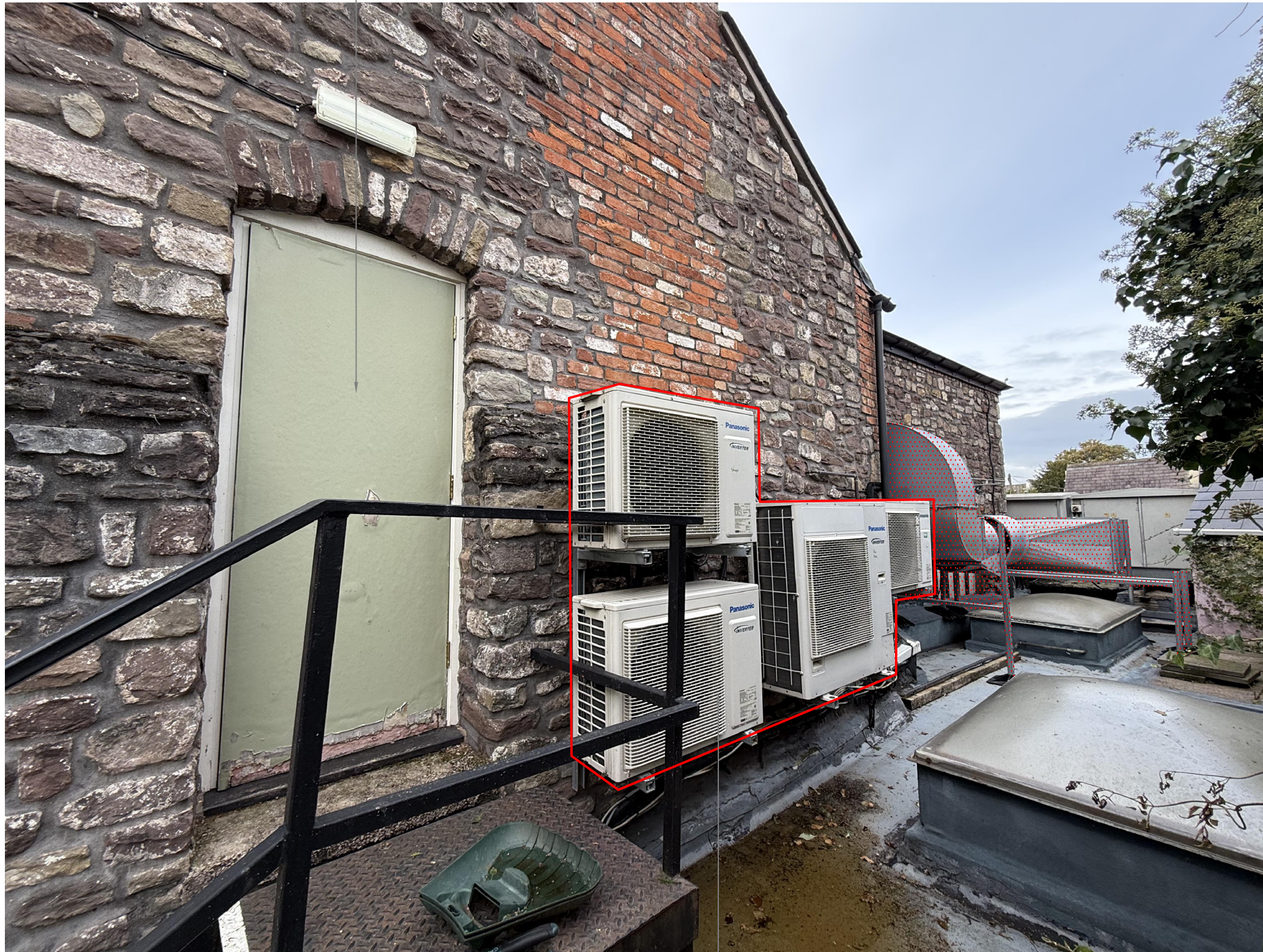
EXISTING LOCATION REFERENCE IMAGE 03 VIEW FROM FLAT ROOF (FIRST FLOOR LEVEL)
