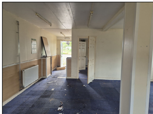
Figure 10 – Glamair Unit Interior, Looking (S)
