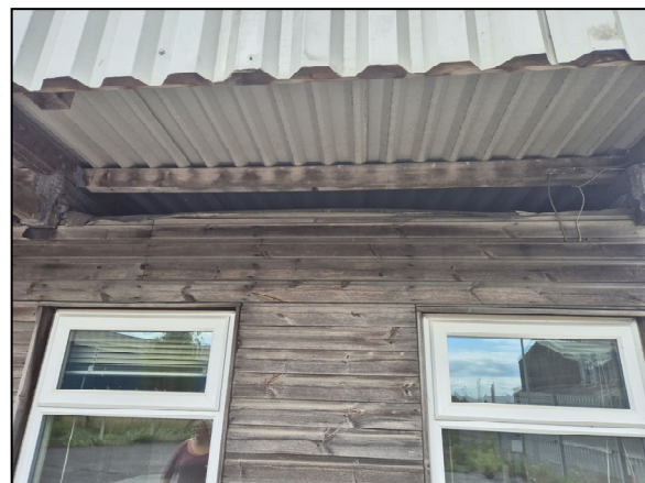
Figure 7 – Gap above Timber Cladding on (S) Wall of Survey Building Enables Access/Egress for Bats to Small Void Located Between the Two ‘Roofs’ of the Building
