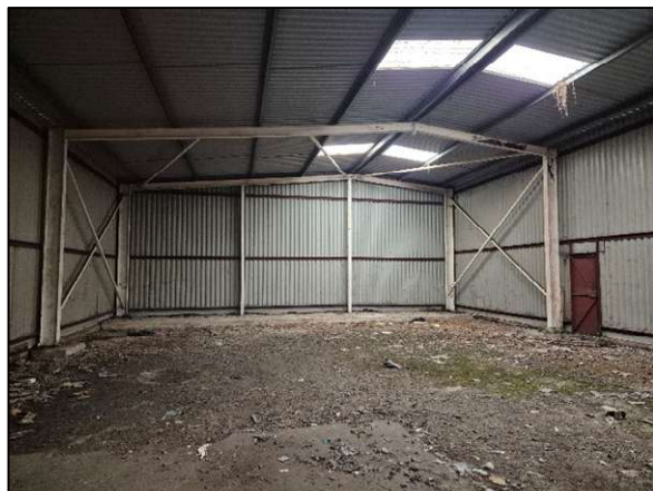
Figure 21 – (W) Steel Clad Wall of Steel Framed Warehouse, Looking (W)
