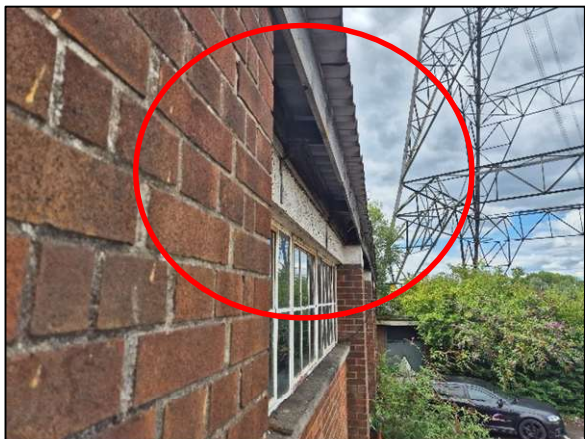
Figure 13 – Gap and Potential Smudging Where Timber Framework Meets Wall in vicinity of Roller Shutter Door at (SE) of Survey Building
