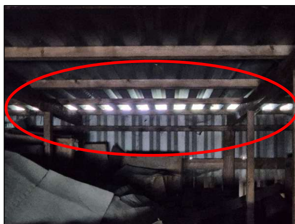
Figure 20 – Light Ingress from Gaps Under Corrugated Roof Sheets May Permit Access/Egress for Bats
