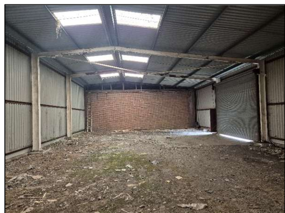
Figure 22 – (E) Brick Wall of Steel Framed Warehouse, Looking (E)
