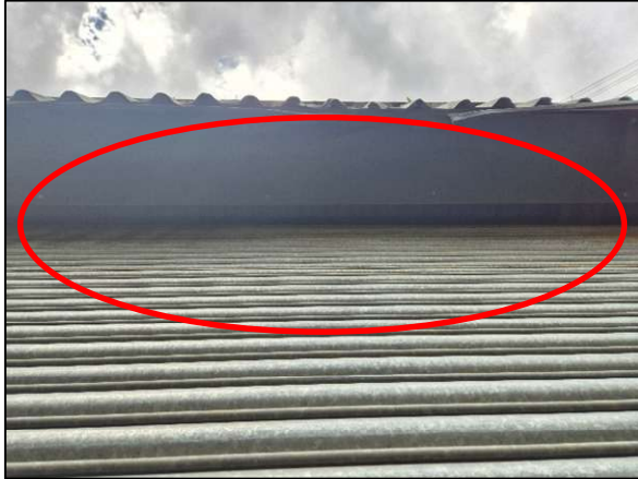
Figure 11 – Gap Behind Timber Fascia Board on (N) Side of Building May Permit Access/Egress for Bats to Interior & Associated PRFs
