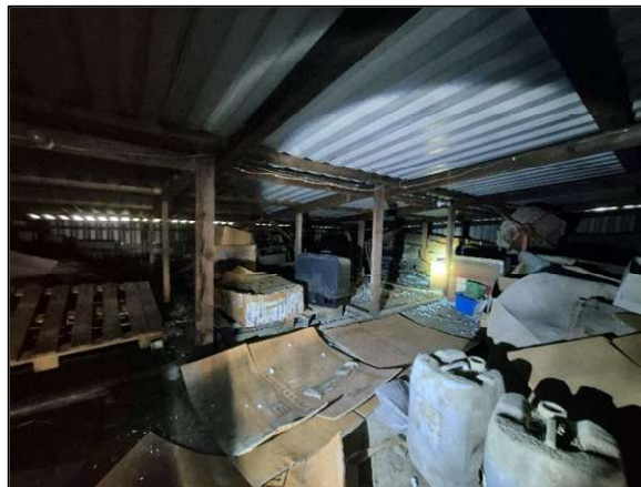
Figure 20 – Light Ingress from Gaps Under Corrugated Roof Sheets May Permit Access/Egress for Bats
