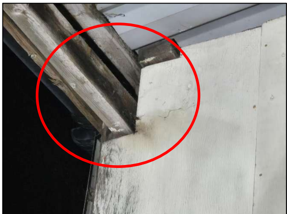
Figure 13 – Gap and Potential Smudging Where Timber Framework Meets Wall in vicinity of Roller Shutter Door at (SE) of Survey Building
