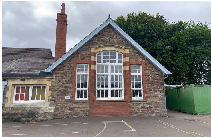
Casement Window NW Elevation
