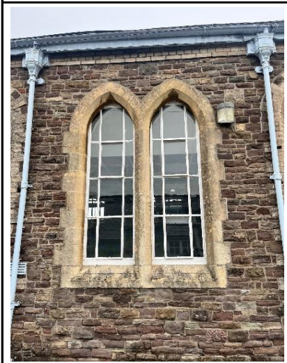
Example bathstone window surround SE Elevation
