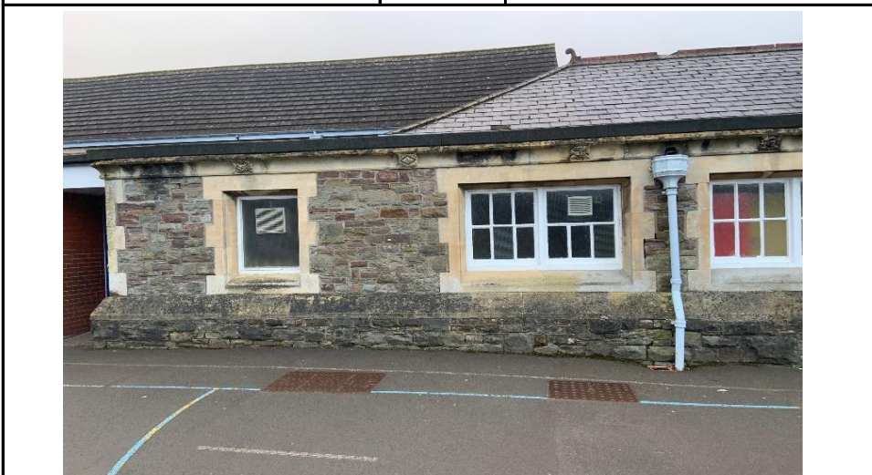
Example bathstone window surround NW Elevation
