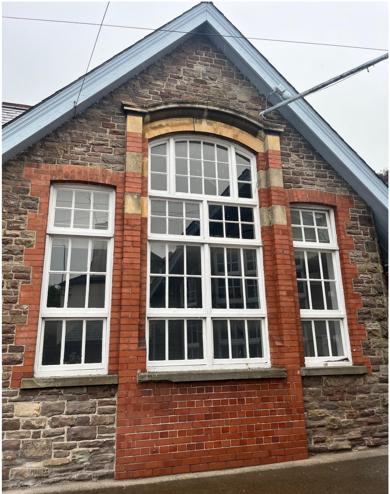
Photo 1: One example of the Casement windows marked for replacement
