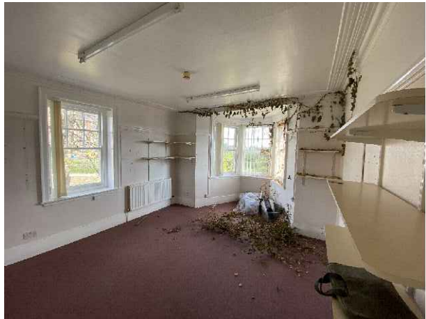
Photo 12: Existing modern type radiator under the window
