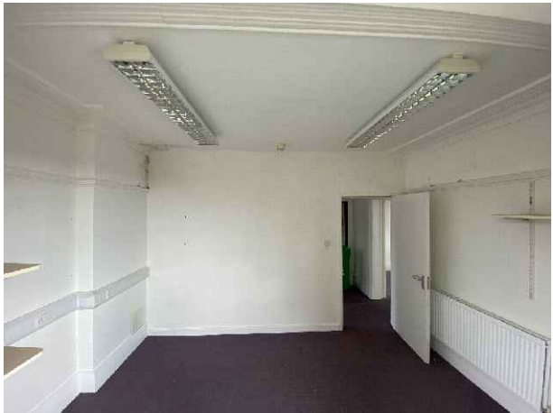
Photo 20: Existing modern type radiator by door
