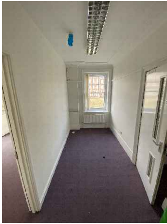
Photo 21: Existing modern type radiator under the window
