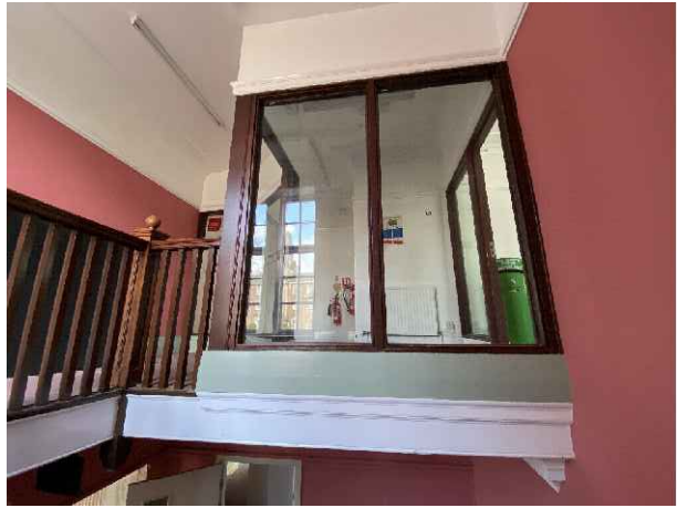
Photo 11: Existing modern type radiator on landing
