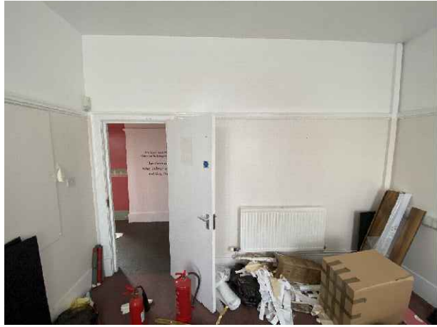
Photo 03: Existing modern type radiator by door
