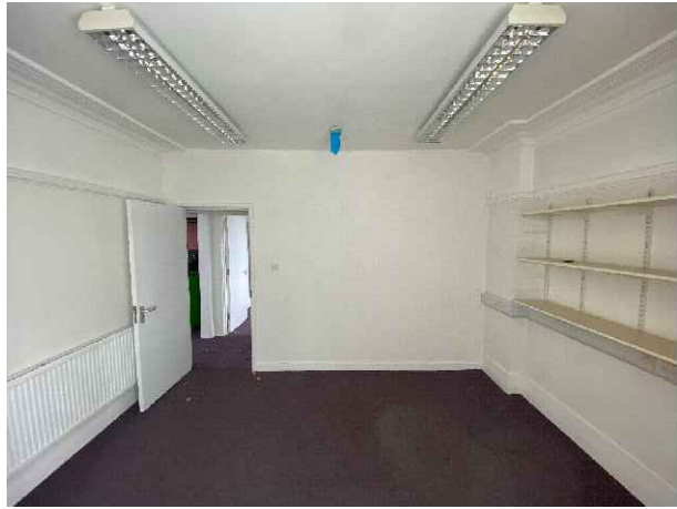
Photo 19: Existing modern type radiator by door
