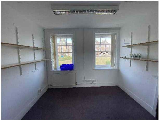
Photo 06: Existing modern type radiator under the window
