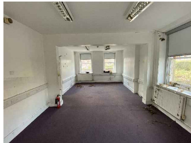
Photo 02: Existing modern type under the window
