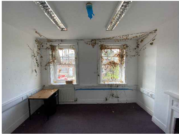
Photo 05: Existing modern type radiator under the window
