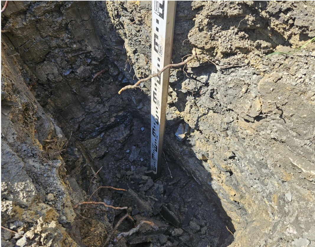
Test 2 – Pit prior to fill.
