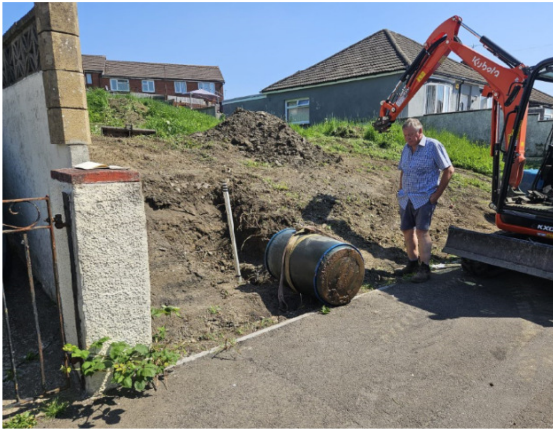
Test 2 – Location, prior to fill.
