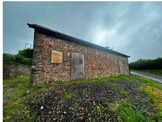
Figure 3.5 – South Eastern Elevation of Barn
