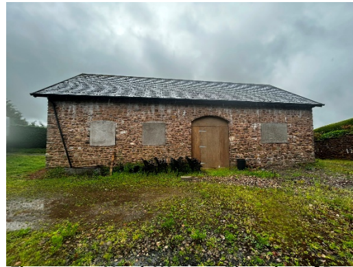
Figure 3.3 – North Western Elevation of Barn
