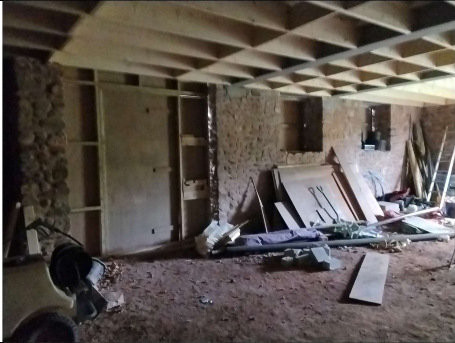
Photo 9. First floor room.
