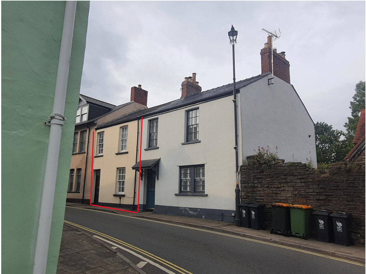
South Elevation, High Street view from south (17 High Street highlighted in red)
