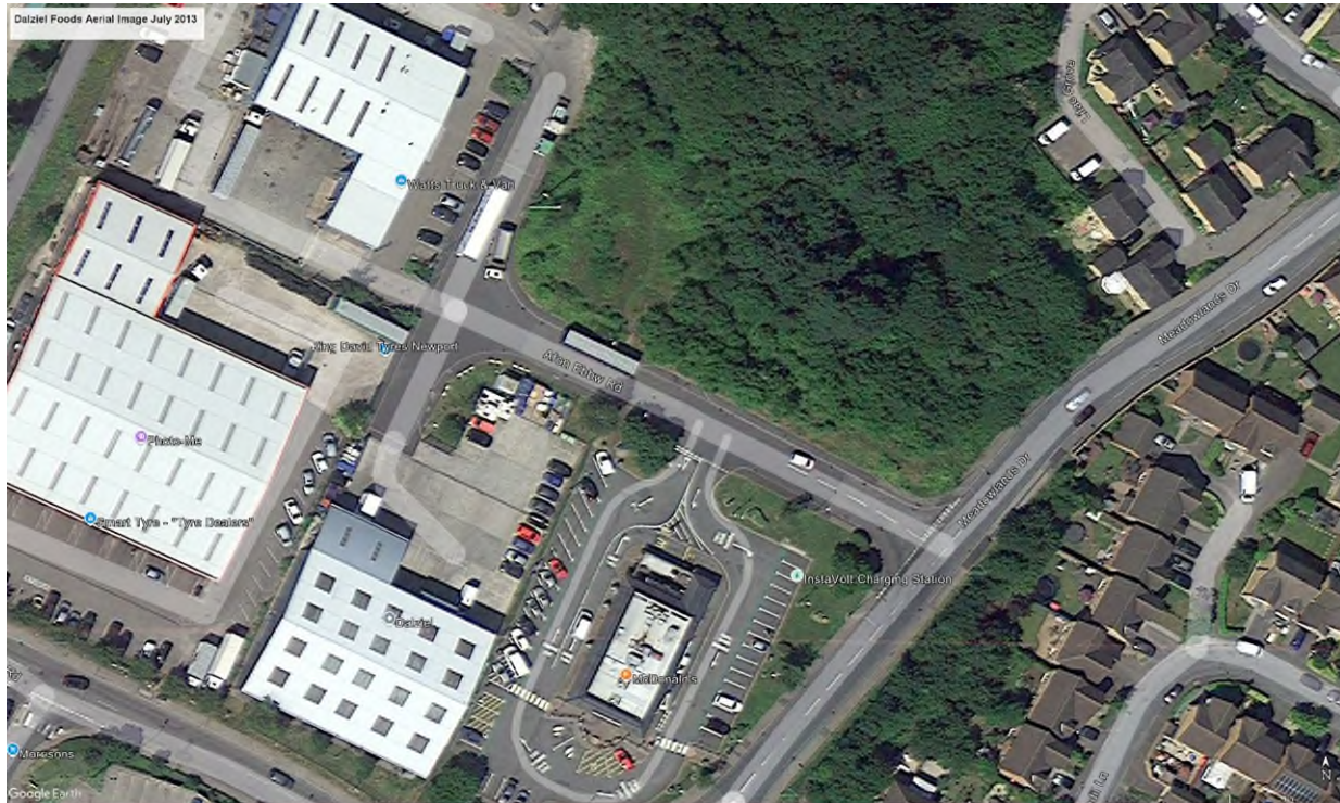
Figure 4: Aerial View of site in 2013
