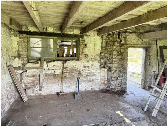
Plate 7. Interior of the stone outbuilding showing heavy historic timber floor beams overhead, a small C20 inserted timber window opening (left, to the north inboard wall), and a doorway opening (right) leading out. Wall fabric shows historic stone walling with brick repairs and patching. The carcassing visible above is to be replaced (see paragraph 7.7).
