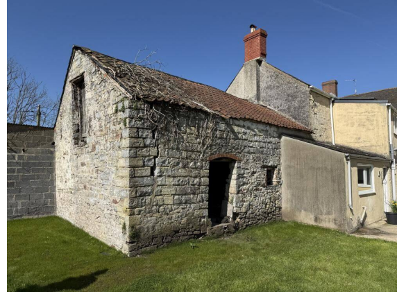
Plate 6. Stone outbuilding (Element 3) from the south-east, showing the existing pantile rear (east) slope and south stone gable. The new roof is to be slate to both slopes (see paragraph 7.6).
