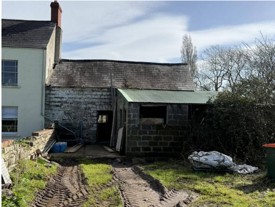
Plate 1. Stone outbuilding (Element 3) viewed from the north, showing the slate front (west) slope. The C20 concrete-block shed (Element 4, corrugated metal roof, to be demolished) abuts on the right with the principal farmhouse beyond.
