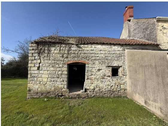
Plate 3. Rear (east) elevation of the stone outbuilding (Element 3), showing the original low arched stock doorway with brick voussoir arch. This position is to form the new bi-fold door opening serving the ancillary accommodation (see paragraph 7.4). The corresponding arched doorway on the west (principal) frontage is to be retained in situ with a recessed infill behind the voussoirs.
