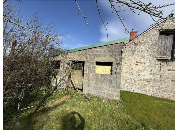
Plate 2. The C20 concrete-block shed (Element 4) abutting the stone outbuilding's north (inboard) wall. Of no listed-building significance; proposed for demolition in its entirety.
