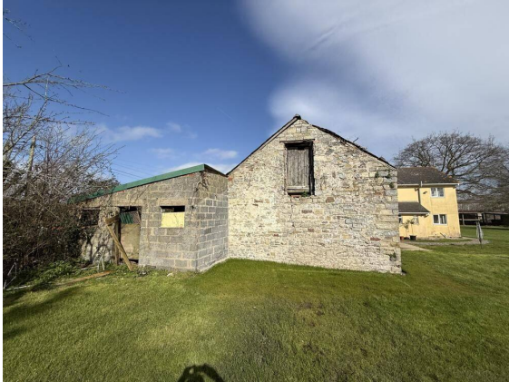
Plate 5. North gable of the stone outbuilding, showing the timber loading opening with the remains of a timber lintel — diagnostic evidence of the original byre or stable function with hayloft.
