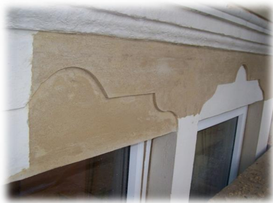
Repair Finished with Mortar Mix
