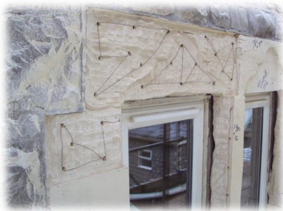
Repair during Reconstruction
