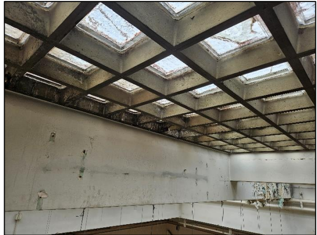
Photograph 4 – Showing section of Glass Rooflight
