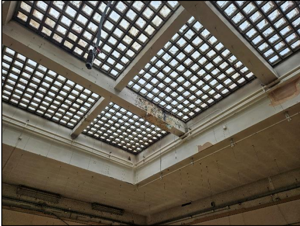
Photograph 1 – View of Rooflight
