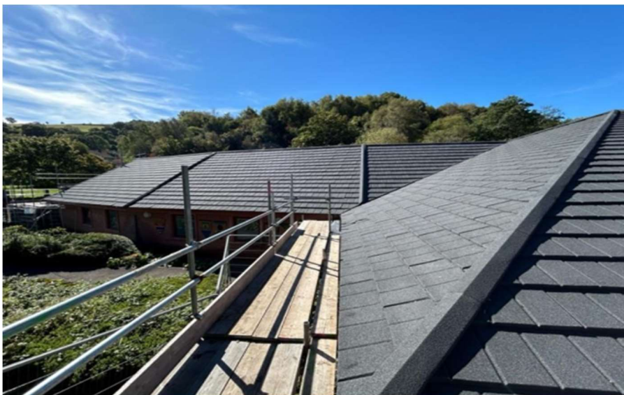
image of a new roof being installed using airtile
