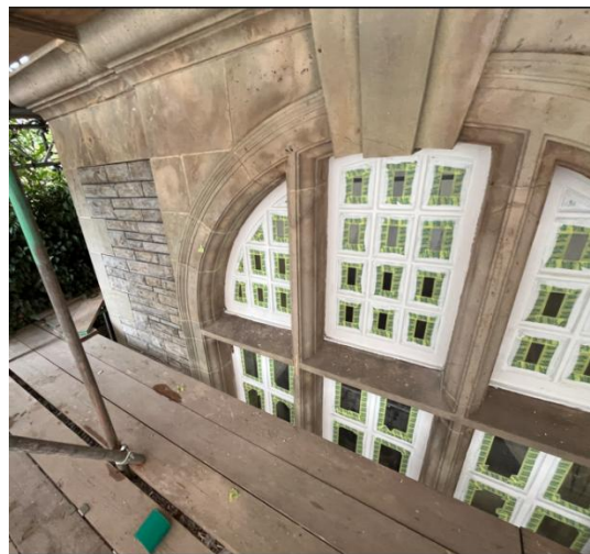
Plate 5: Window W01 Following steam cleaning
