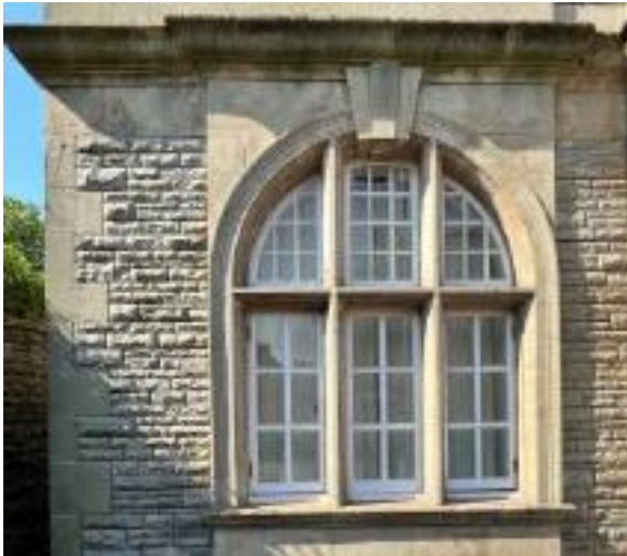
Plate 4: Window W01 Prior to steam cleaning
