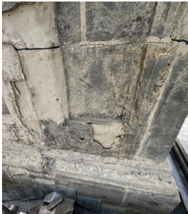
Plate 1: Existing pointings (chimney 5) soft sand / washed sharp sand)
