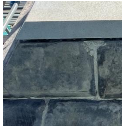
Plate 2 & 3: Trial sections of stone repointing (1:3:1 NHL2.5 /
