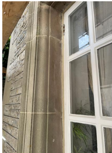
Plate 5: Window W01 Following renewed pointings
