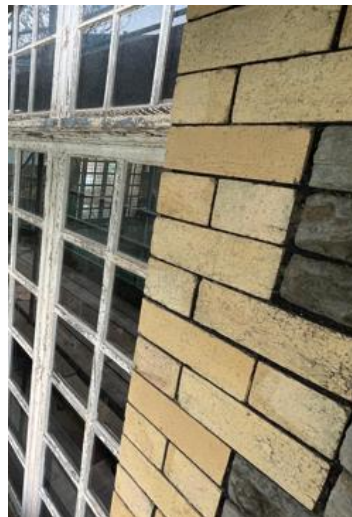
Plate 4: Trial sections of repointing to brickworks (1:3:1 NHL2.5 / Blaenavon Dark / washed sharp sand)
