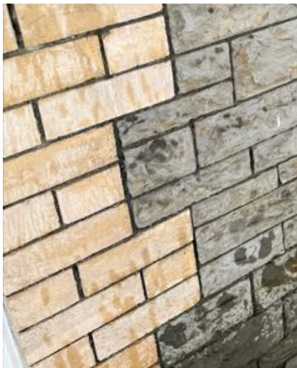
Plate 3: Existing yellow stock brick pointings
