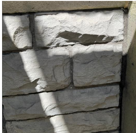
Plate 2: Trial sections of stone repointing (1:3:1 NHL2.5 / Blaenavon Dark / washed sharp sand)
