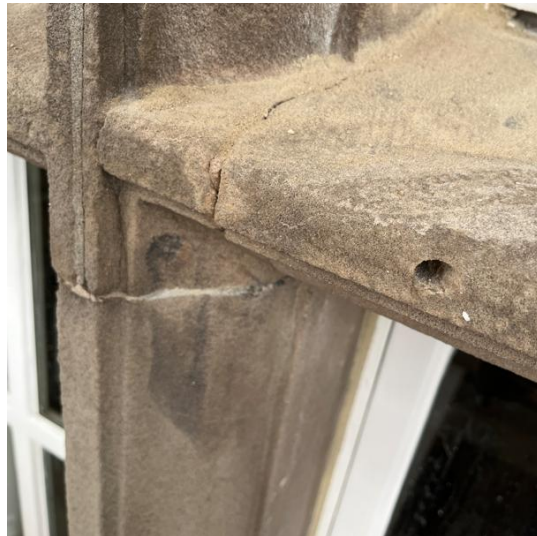
Plate 2: Trial sections of stone stitching to stabilise transom crack / parting.
