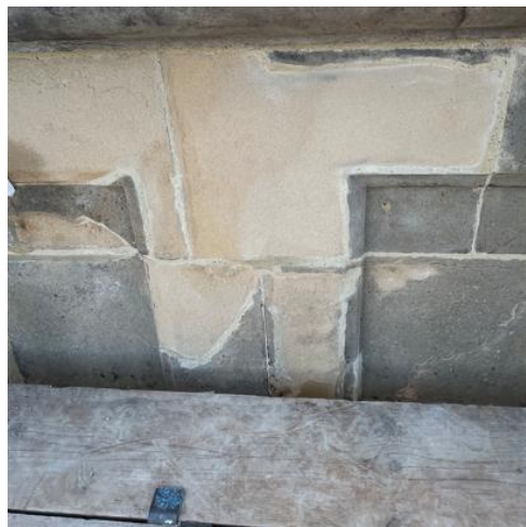
Plate 2: Trial sections of stone stabilisation / shelter (Apply behind delaminations and to all cleaved edges to re-bond. NHL 3.5; washed sharpsand; Natural goat hair 1:3:1 ratio)
