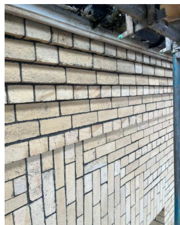
Plate 3 & 4: application of clear Keim Lotexan product on site to existing stones and brickworks.
