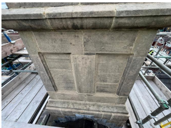
Plate 3 & 4: application of clear Keim Lotexan product on site to existing stones and brickworks.
