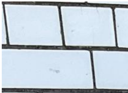
Plate 2: repaired and repointed ceramic brick
