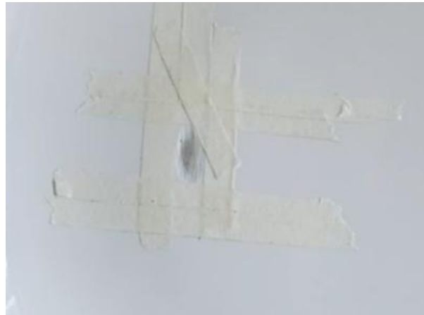
Plate 3 & 4: Application of off white polyester resin repair to ceramic bricks on site
