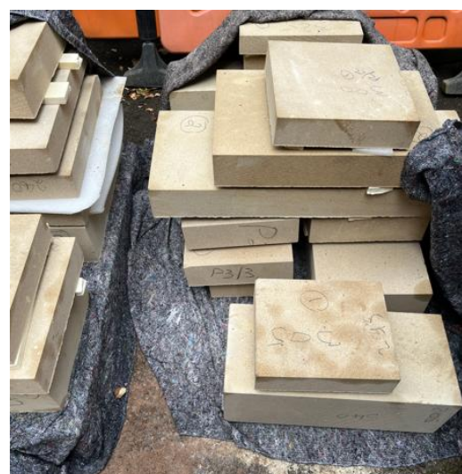
Plate 4: New stone arrived ready for carving
