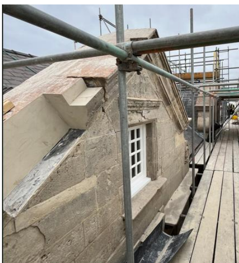
Plate 3: Cutting out defective stones
