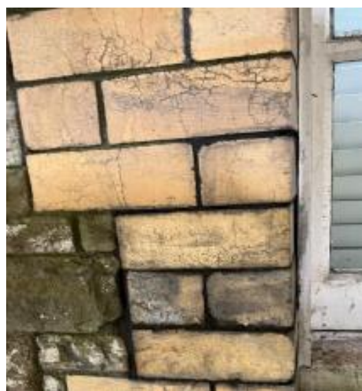
Plate 4: repair of bricks
