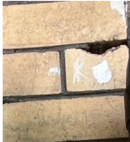
Plate 2: Careful removal of ironmongery
