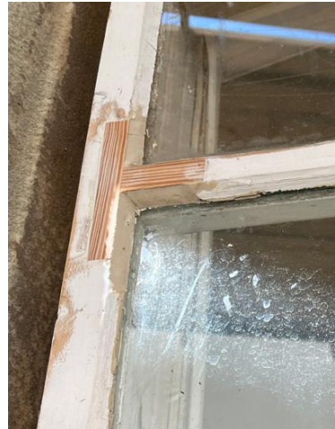
Plate 4: scarfed timber repair made
