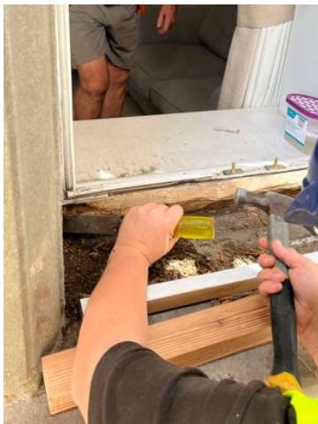
Plate 3: Cutting out rotten timber
