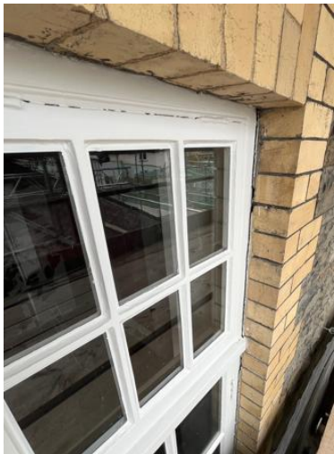
Plate 3: Replacement glazing pane
