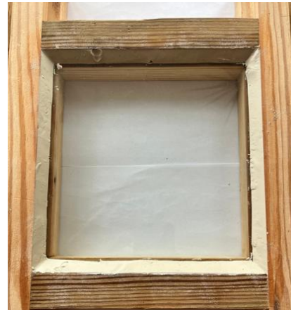
Plate 2: New LINSEED oil traditional putty
