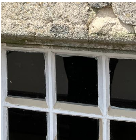
Plate 3: On site fitted and new putties applied
