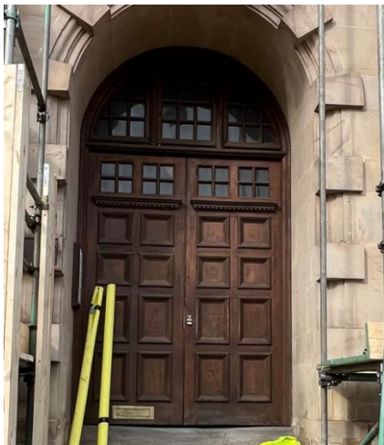
Plate 1: Existing doors / fanlight to front elevation
