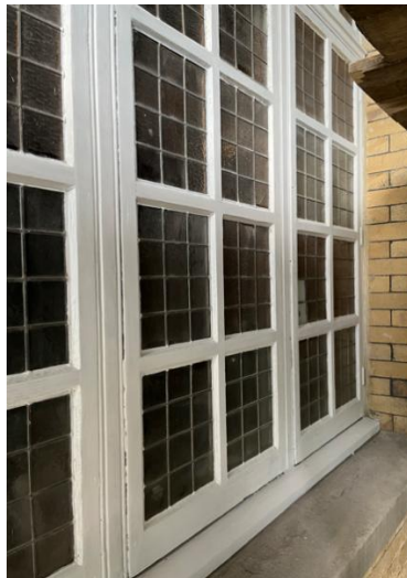
Plates 3,4 & 5: Windows and external joinery decorated on site with Little Greene, Toms' old oils Colour / Type to be: Loft White Eggshell oil based paint.
