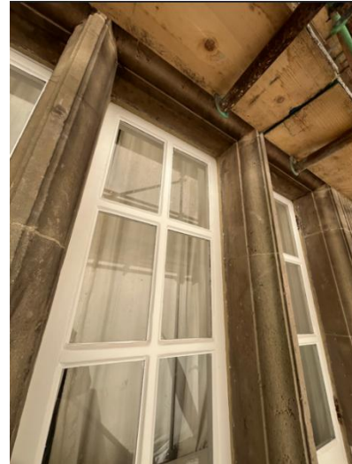
Plates 3,4 & 5: Windows and external joinery decorated on site with Little Greene, Toms' old oils Colour / Type to be: Loft White Eggshell oil based paint.
