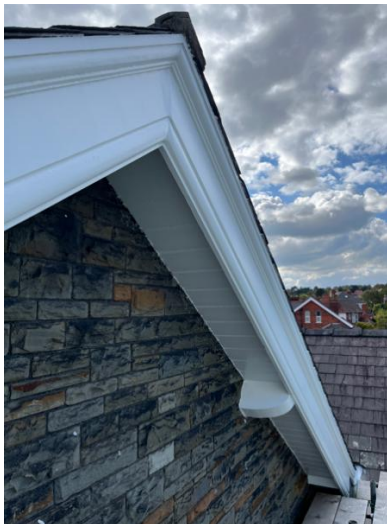
Plates 3,4 & 5: Windows and external joinery decorated on site with Little Greene, Toms' old oils Colour / Type to be: Loft White Eggshell oil based paint.
