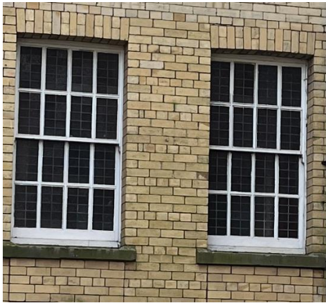
Plate 1: Existing windows prior to decorating
