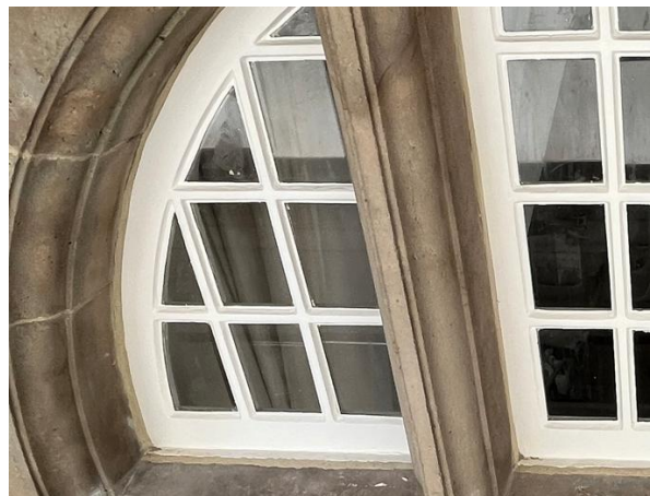
Plate 2: New lime mortar edge seal installed
