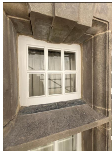
Plate 2: New lime mortar edge seal installed
