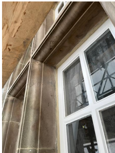
Plate 1: Defective Lime edge seals carefully removed
