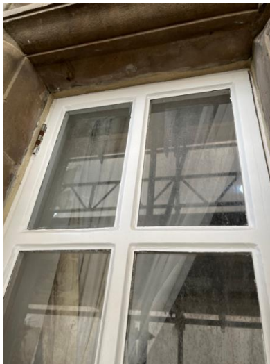
Plate 1: Defective Lime edge seals carefully removed
