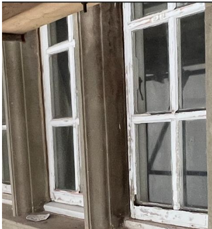
Plate 1: Defective Lime edge seals carefully removed
