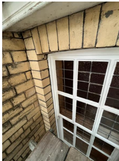
Plates 3,4 & 5: Selection of windows to subservient façades (all windows and doors within brick reveals to receive) proposed renewed silicone edge seals to be installed (matched closely to existing and masking of bricks to be completed prior to application to prevent over application to bricks).
