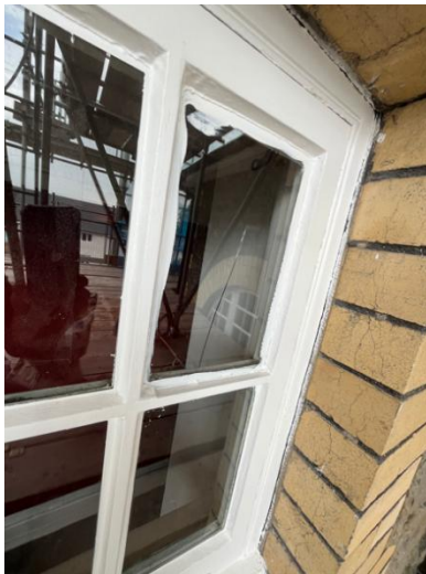
Plates 3,4 & 5: Selection of windows to subservient façades (all windows and doors within brick reveals to receive) proposed renewed silicone edge seals to be installed (matched closely to existing and masking of bricks to be completed prior to application to prevent over application to bricks).
