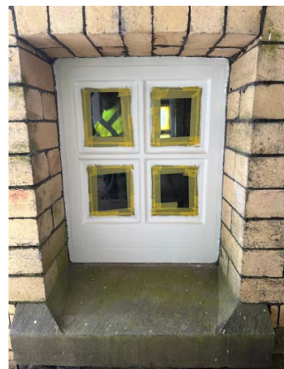
Plates 3,4 & 5: Selection of windows to subservient façades (all windows and doors within brick reveals to receive) proposed renewed silicone edge seals to be installed (matched closely to existing and masking of bricks to be completed prior to application to prevent over application to bricks).
