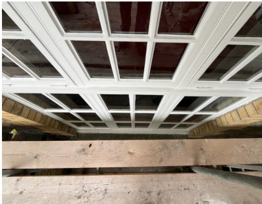
Plate 1: Defective silicone seals carefully removed. Plate 2: New white silicone edge seal PROPOSED.
