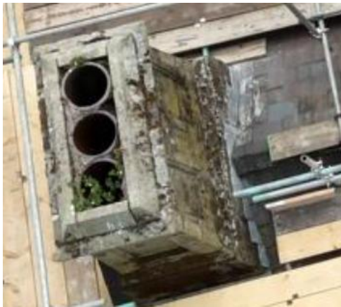
Plate 1: Chimney prior to capping.
