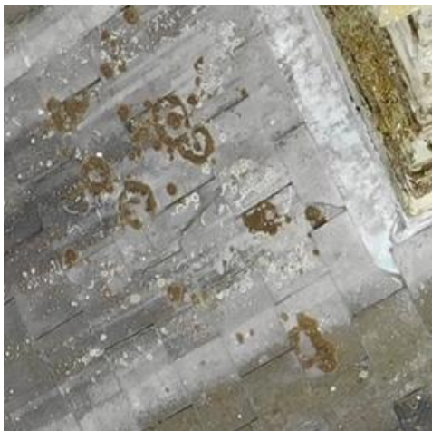
Plate 1: Existing defective slates
