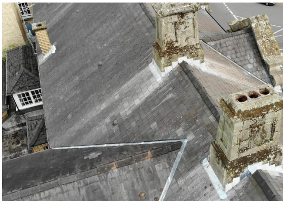
Plate 1: Existing defective slates
