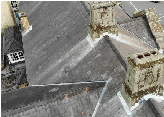
Plate 1: Existing defective ridge tiles
