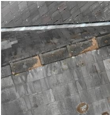
Plate 1: Existing defective ridge tiles
