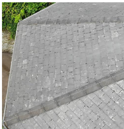
Plate 2: Matched Marley clay ridge tiles to replace
