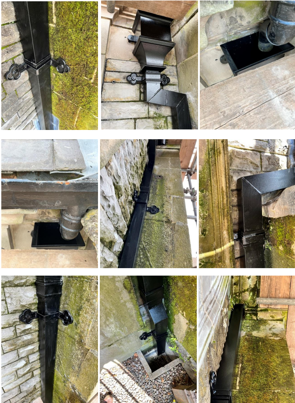
Plates 3-11: Replaced rainwater goods to Bay 5, Front façade (replaced in 2023).
