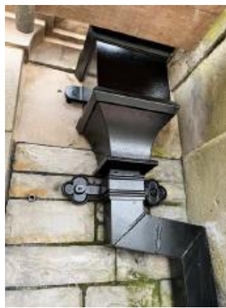
Plate 2: Previously replaced rainwater goods (Bay 5)
