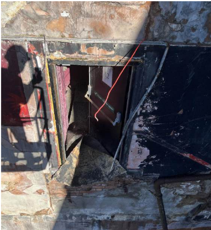
Photo 12 – Showing high level fire escape door.
