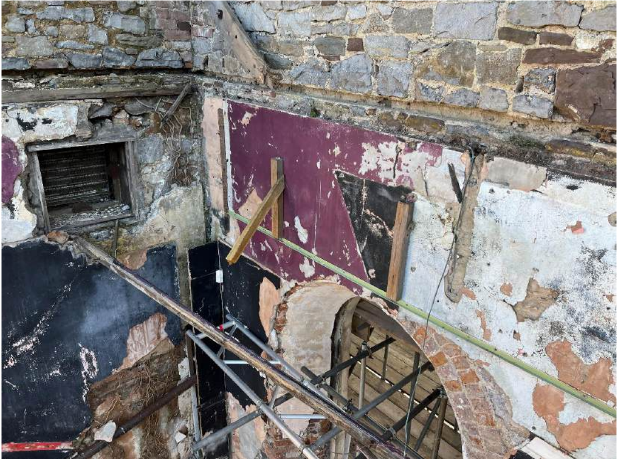
Photo 24 – Showing corner of elevation 1 and 2a
