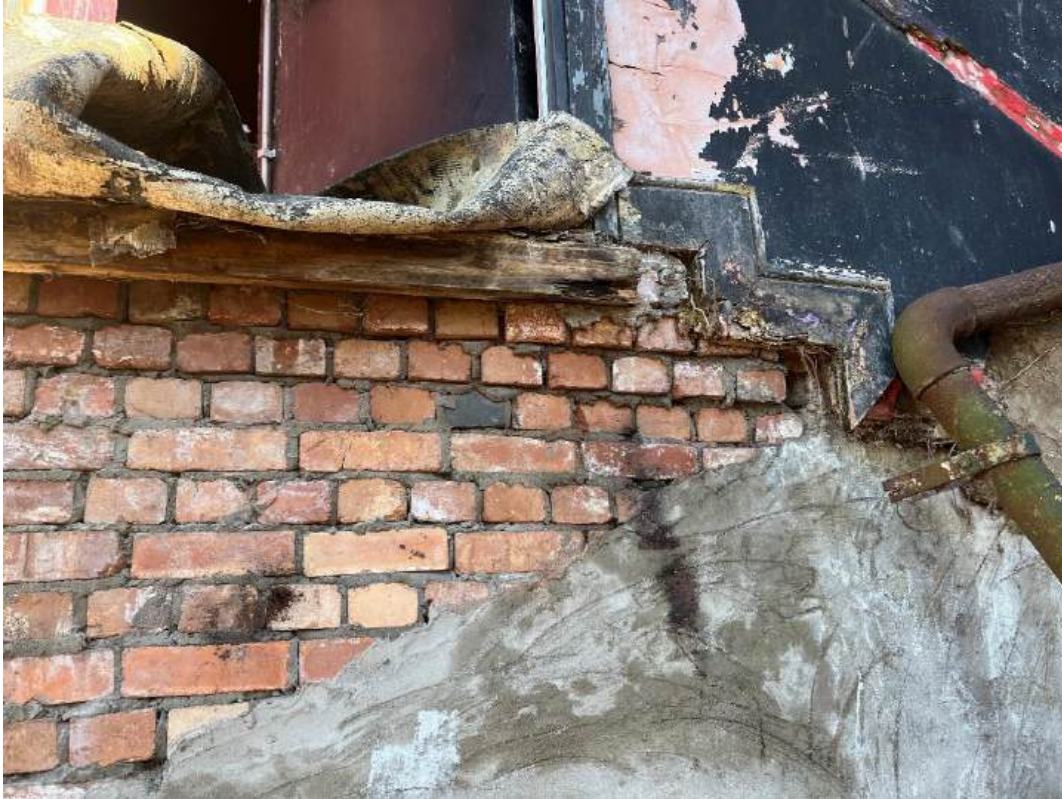
Photo 11 – Showing timber door threshold and stair profile.
