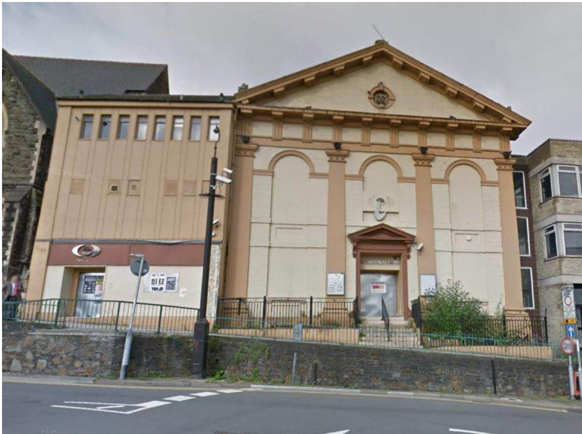
Photo 02 – Showing the front elevation of Zanzibar (from Google Maps Aug 2012).
