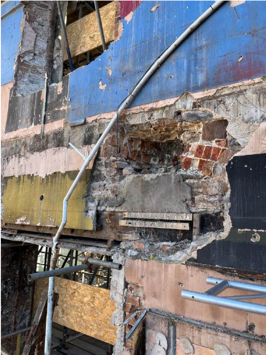
Photo 19 – Showing main entrance doorway
