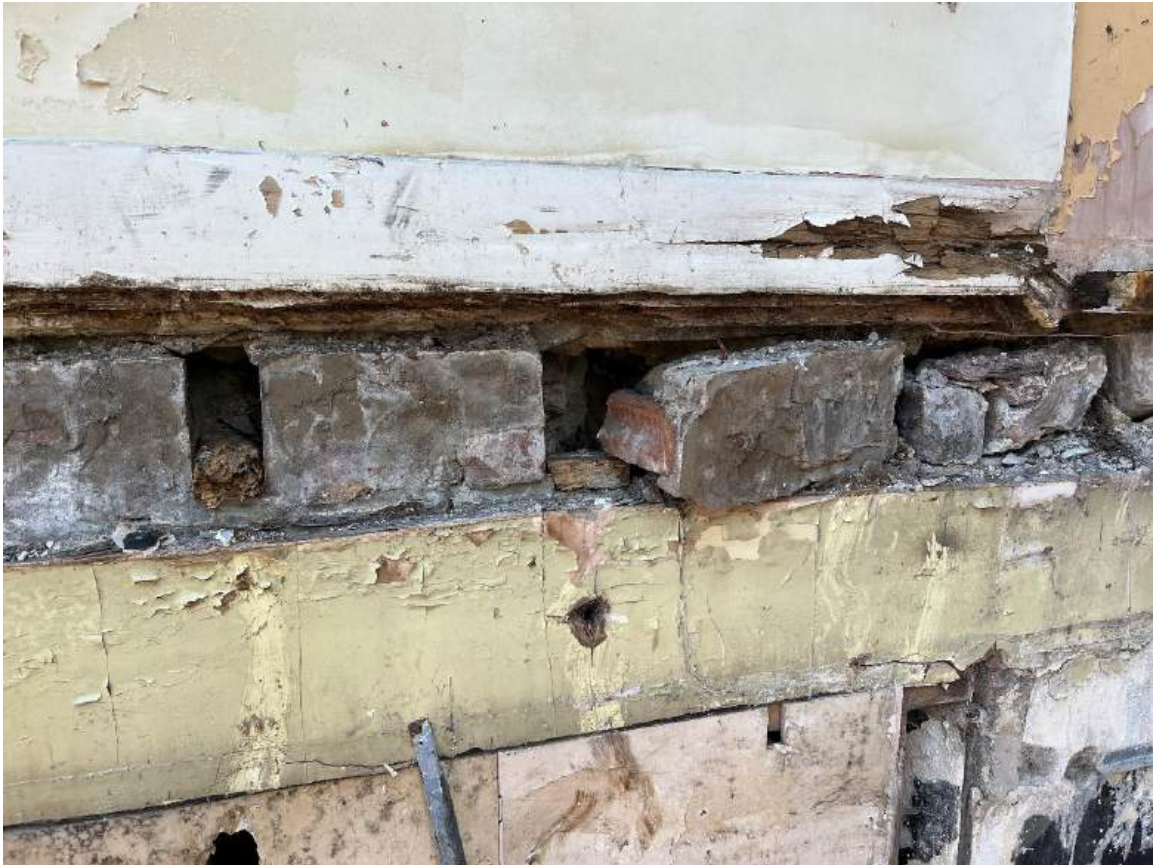
Photo 07 – Showing ground floor level timber floor notches in wall.
