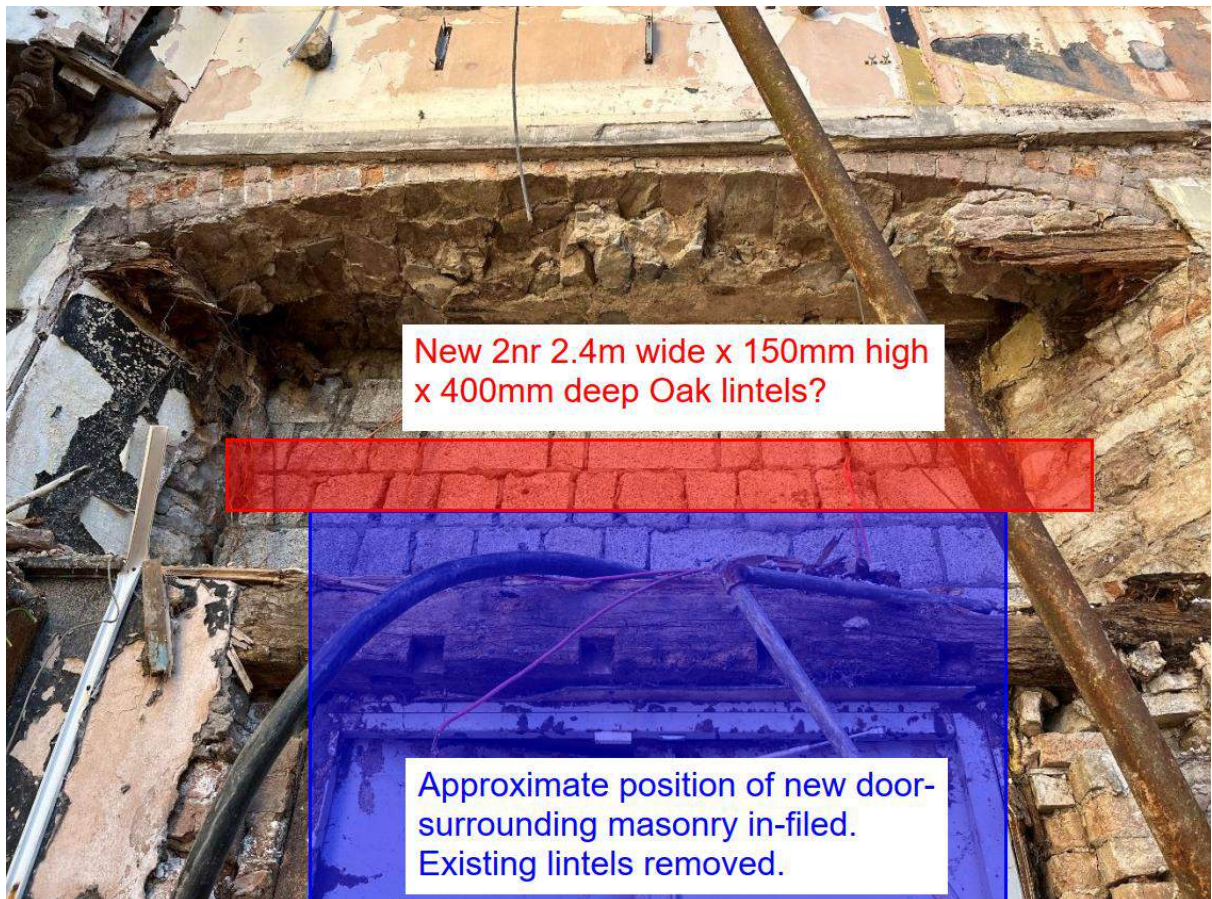
Photo 17 – Showing underside of brick arch
