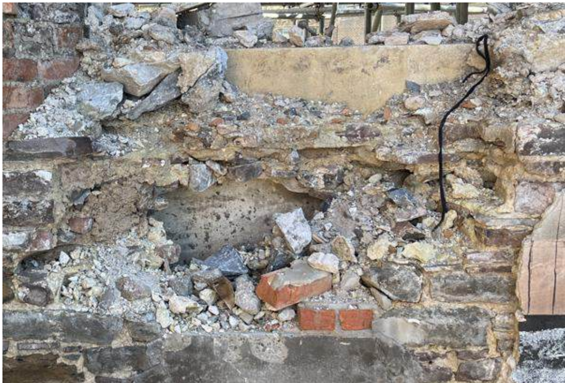
Photo 36 – Showing opening in stone façade
