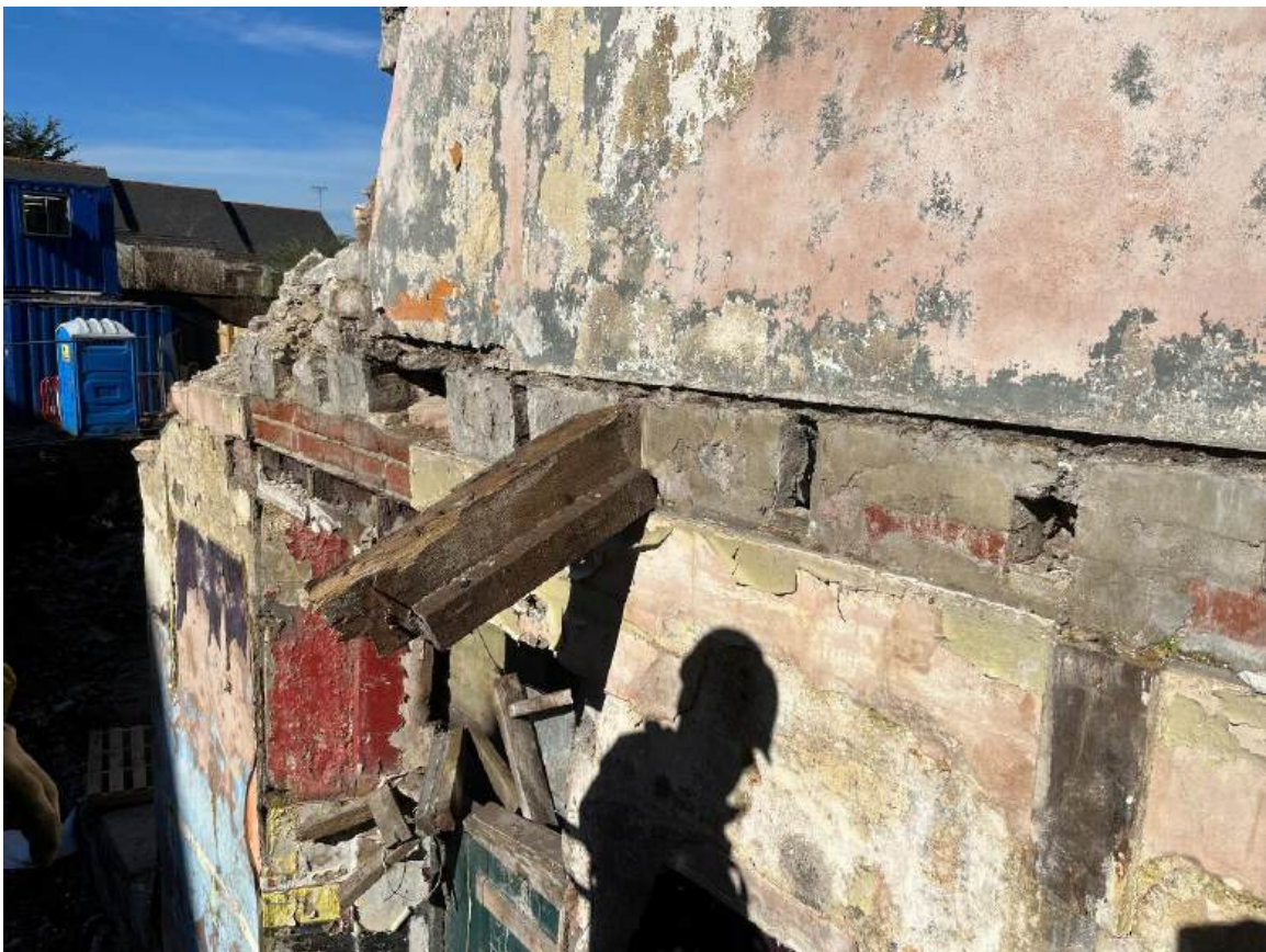
Photo 08 – Showing ground floor level timber floor notches in wall.
