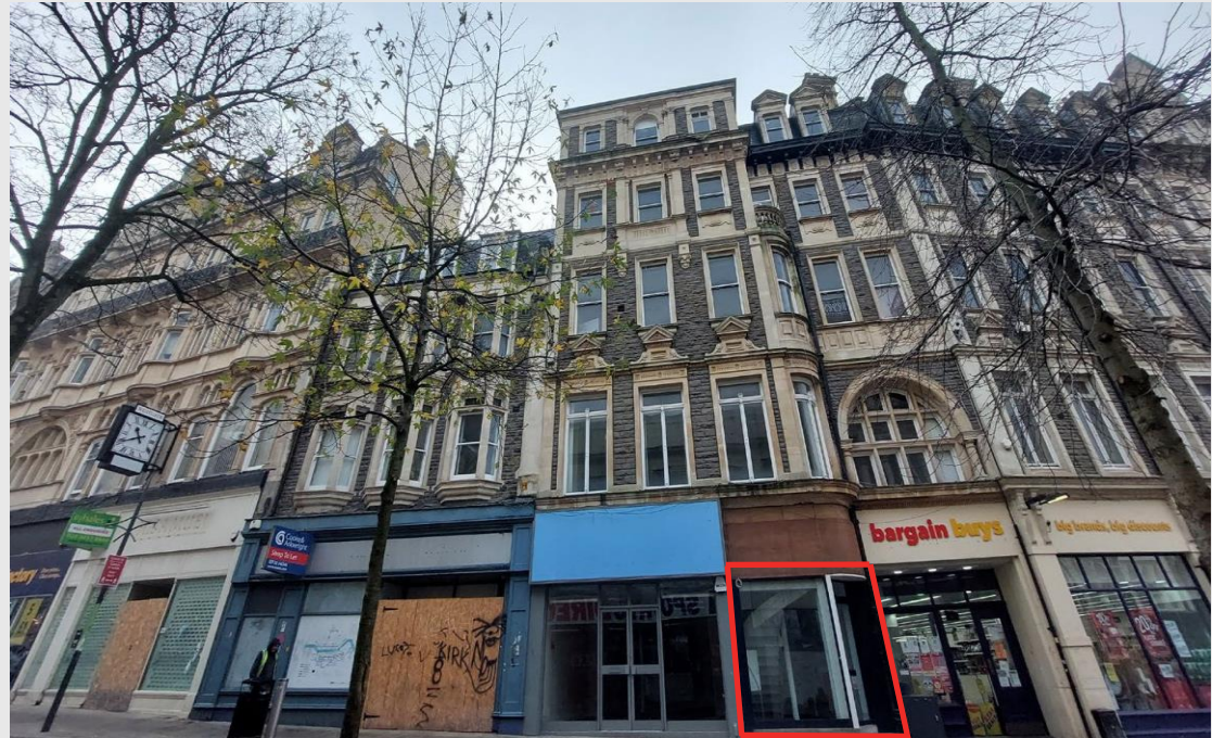
Fig. 1 - Main entrance to the building marked in red.
