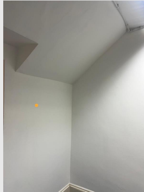
Fig 4- Showing load bearing wall with stairs springers marketed with orange point
