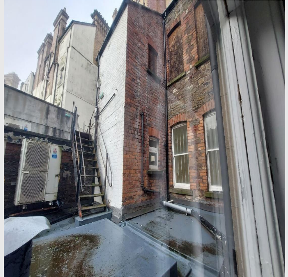
Fig 11 - View of the courtyard to the rear of Unit 3, depicting existing soil vent pipes and downpipes.
