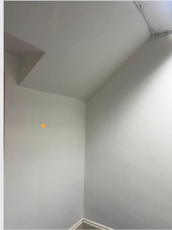
Fig 7- Showing load bearing wall with stairs springers marketed with orange points
