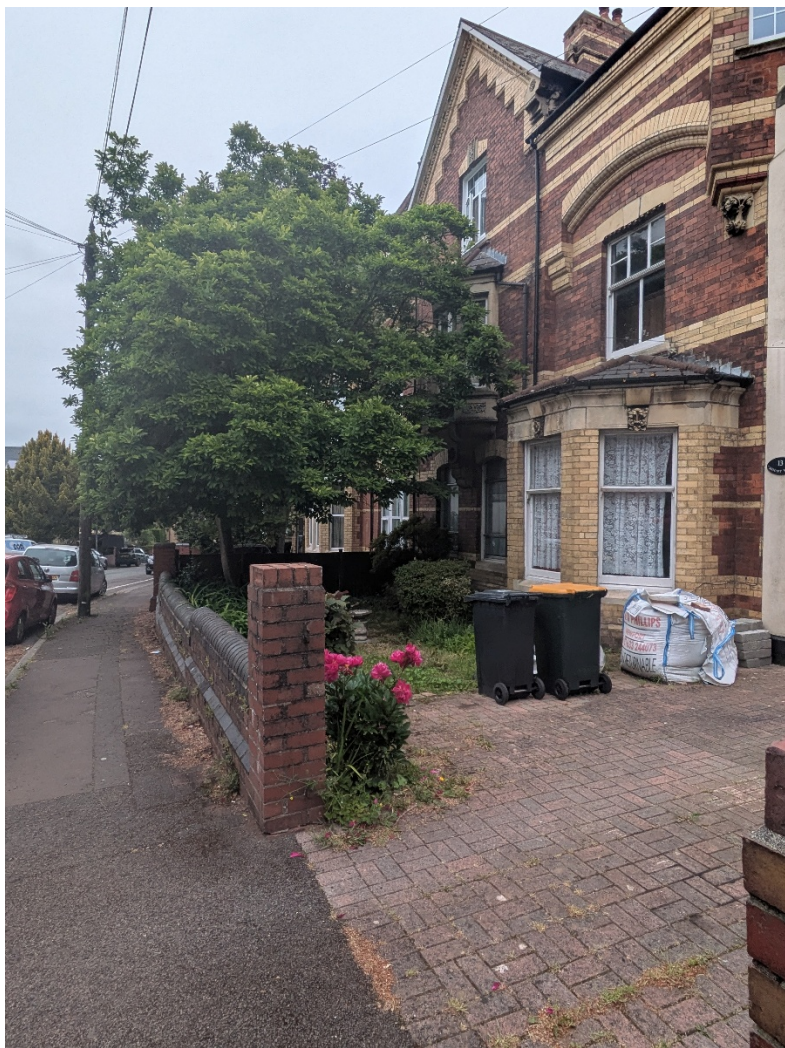
Site plan photos – shows location of tree to front of property
