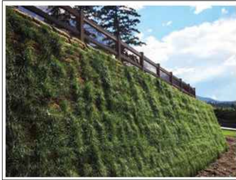
AFTER HYDROSEED AND ESTABLISHED
