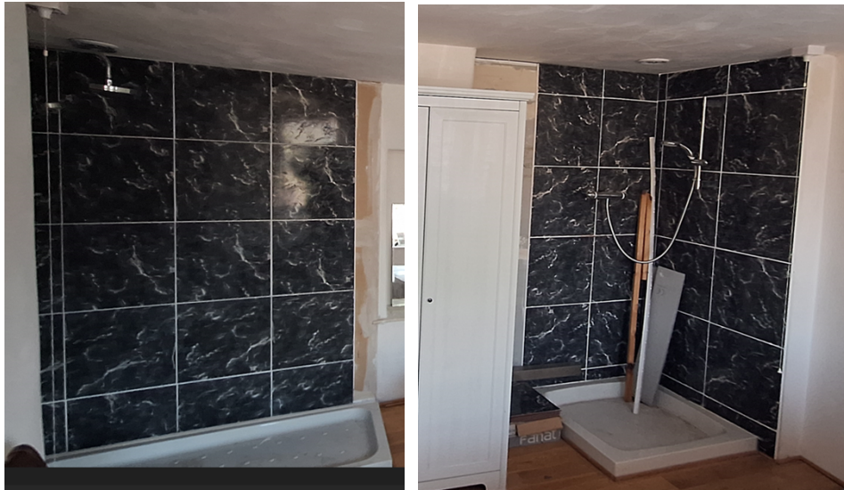
Fig 8 & 9 Partially Completed Bathrooms
