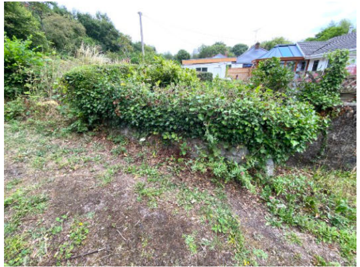
Stone wall either side of track where small stream passes under entrance track
