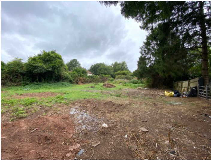
View north across the site from the south east corner of the site, showing cleared areas
