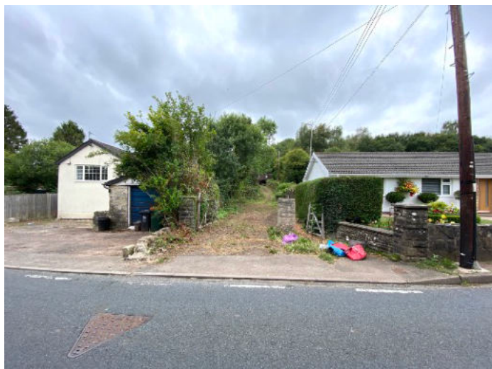
Site entrance track, viewing west from Catsash Road
