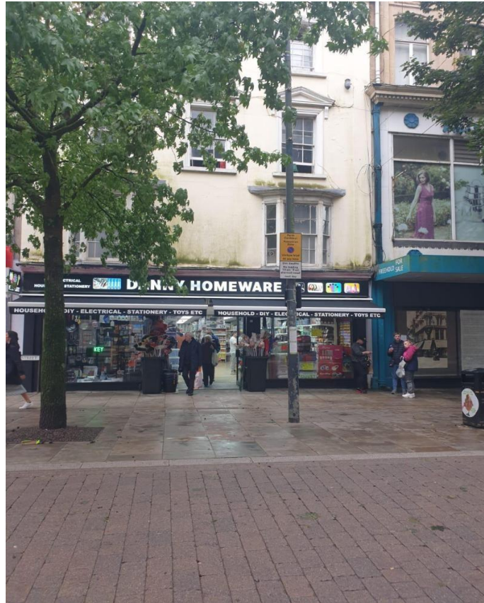
Fig 3: Showing Existing Street view from Commercial Street.
