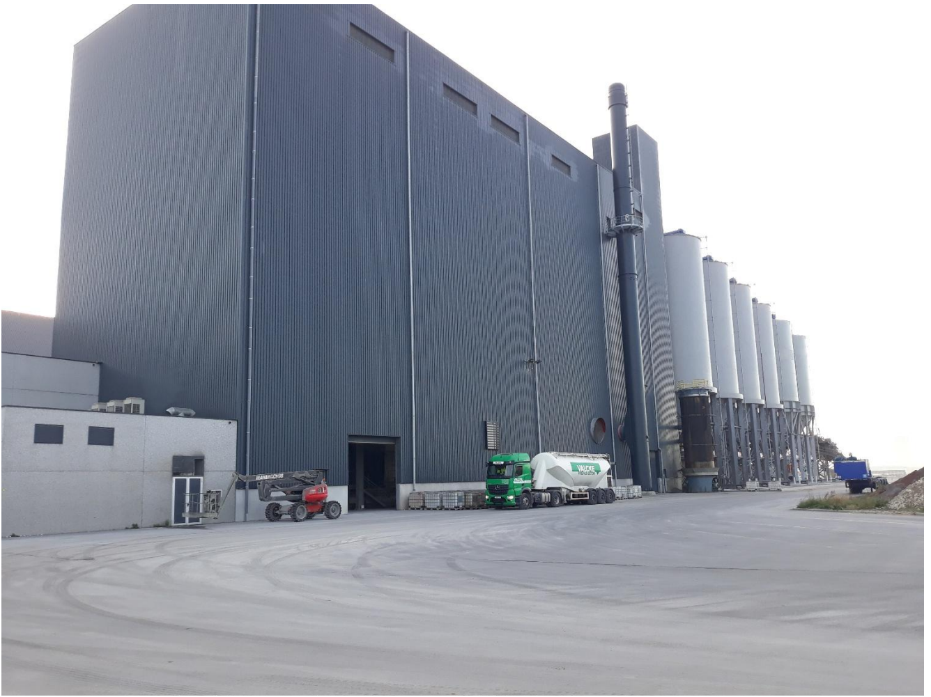
Steel cladding for the façades of the mill building
