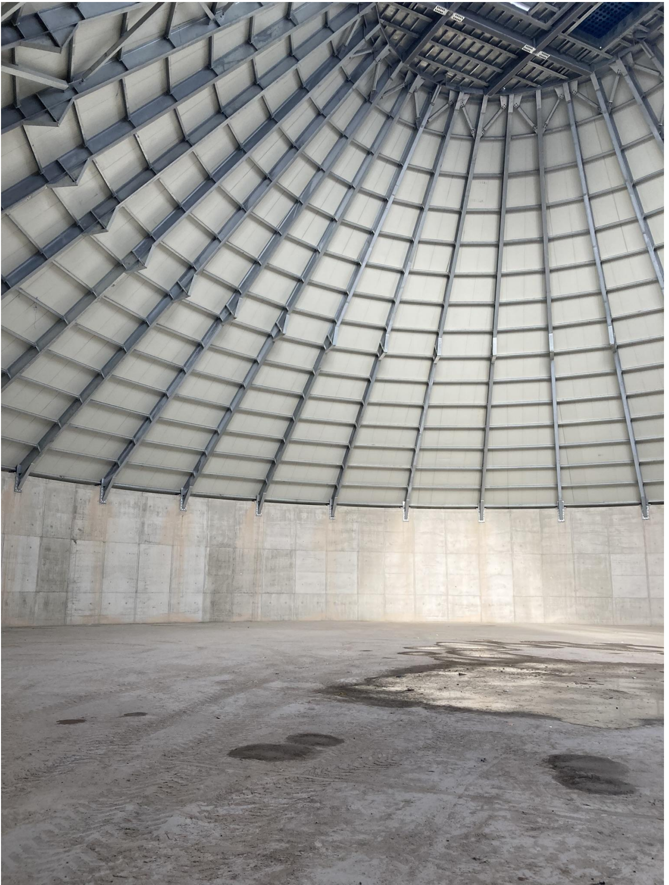
Walls in in situ concrete, structural steel for the roofs, insulated steel cladding for the roof panels
