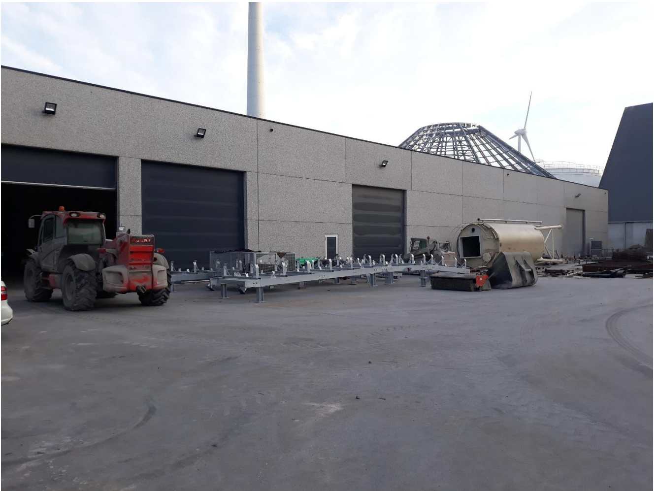
Concrete prefabricated insulated sandwichpanels (washed out finishing) for maintenance warehouse
