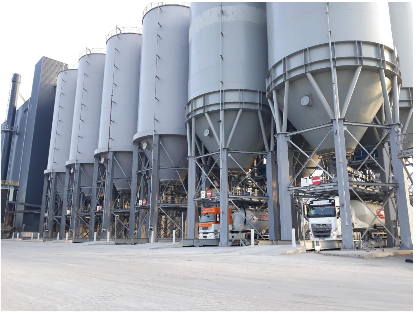
Construction steel and steel silo's
